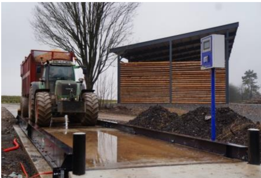
Figure 31. Pont bascule (Source : uvcw)
